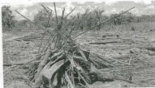
Remains of the demolished house that was being constructed by Miembe Saba Primary School teacher Ayoub Mruthu. The house is said to have been demolished after the Bagamoyo district leadership invaded the school one day after photographs of the house were published in this paper and the leaders are said to have questioned the validity of the house.
